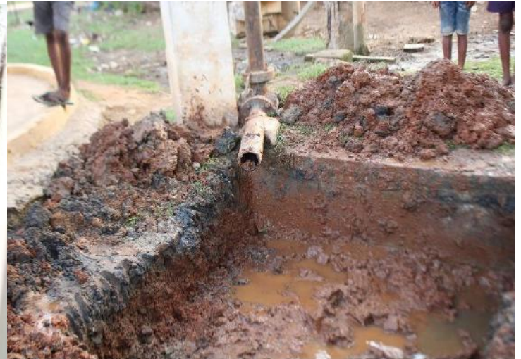
water storage pit near the water tank
